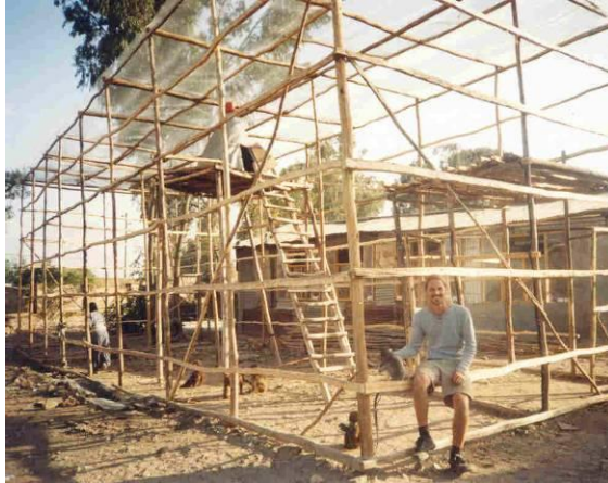
a Canadian volunteer working on the monkey enclosure
